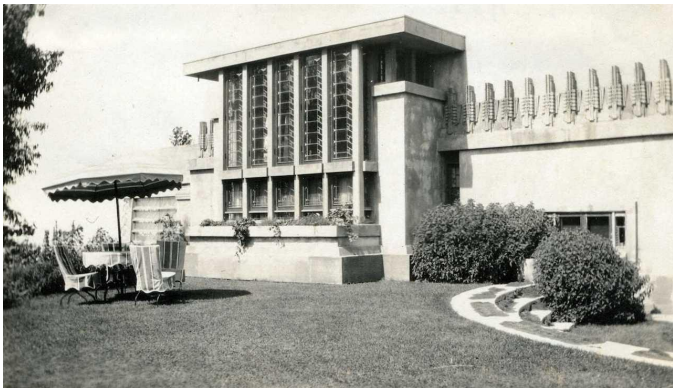
East façade, Hollyhock House. Courtesy of David Devine and Michael Devine. DOWNLOAD THIS PHOTO
